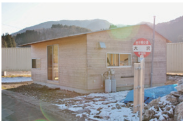
ECO-HOUSE (Ecologically-friendly House) completed in Osawa district. This house is expected to become a communal space accessible to everyone as part of the preparation for moving to higher grounds.
