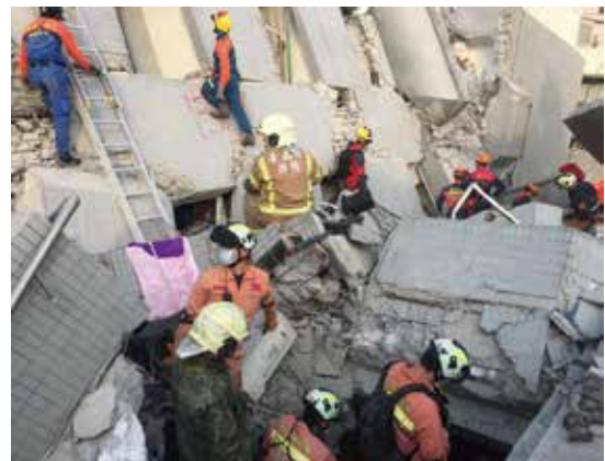
Searching at collapsed buildings
